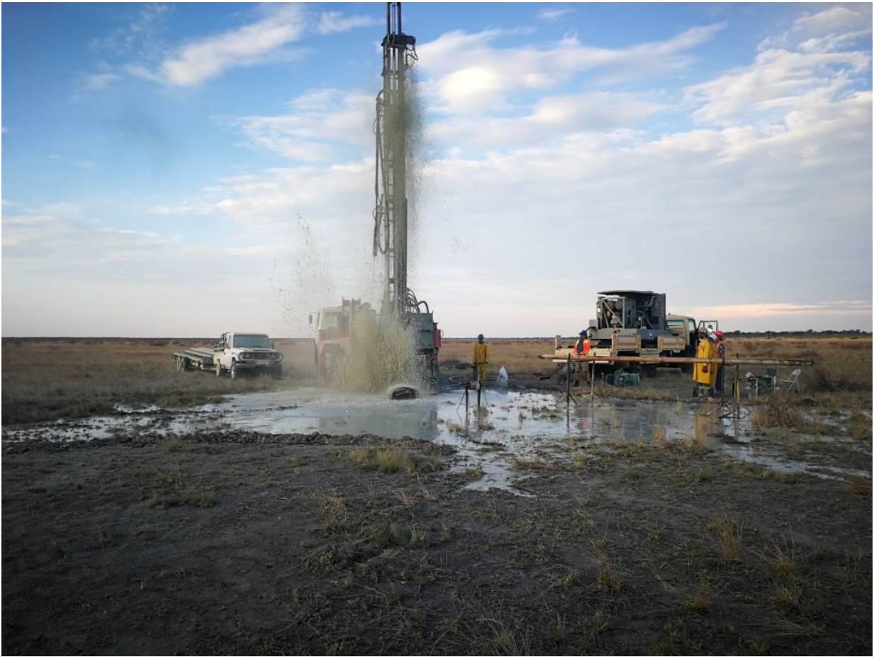
Figure 2: Drilling with strong water strikes
